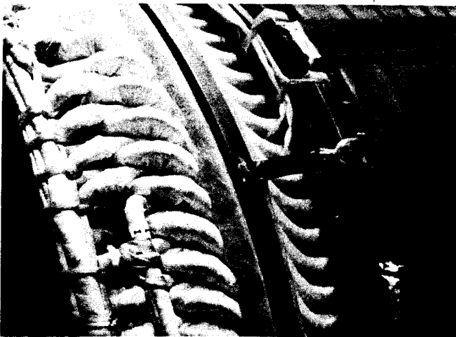
Figure 2. Coil-Lock Bracing Prior to VPI Treatment
